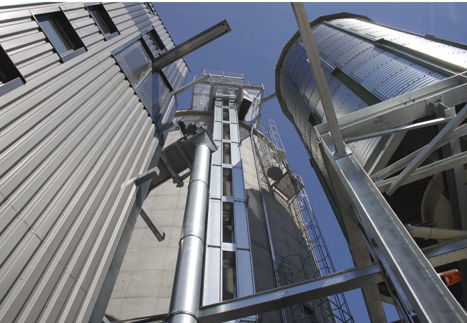
Pellet plant including PELLET.TOWER (left), raw material intake (right), and pellet silo (back)
